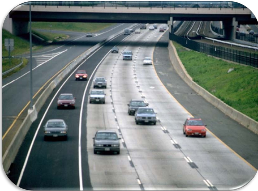
Figure 11. Photo. I-66 HOV/Shoulder Lane Adaptation—Virginia (Photo Courtesy of VDOT).
