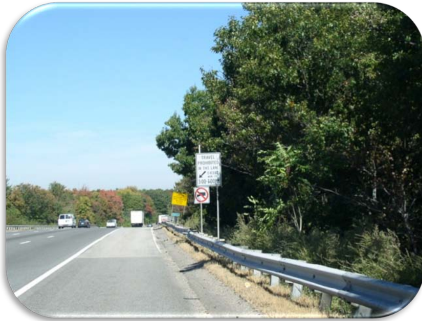
Figure 21. Photo. Regulatory Shoulder Use Signs (Photo Courtesy of MassDOT). (23)
