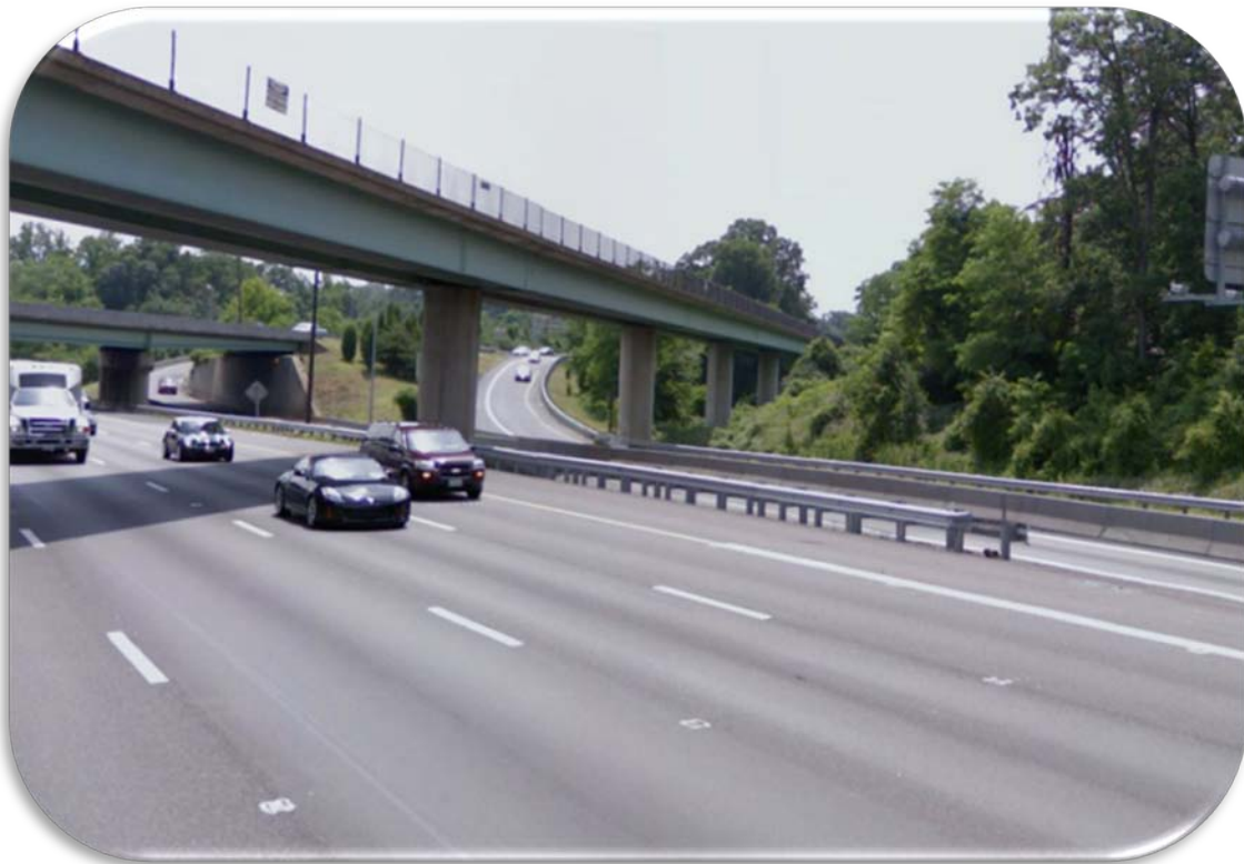
Figure 44. Photo. I-495, Viewing Dual Entrance Ramps from I-66—Virginia.
