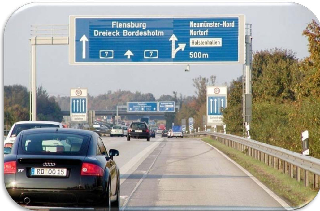
Figure 31. Photo. Continuation of Temporary Hard Shoulder Use through an Interchange—Germany. (13)
