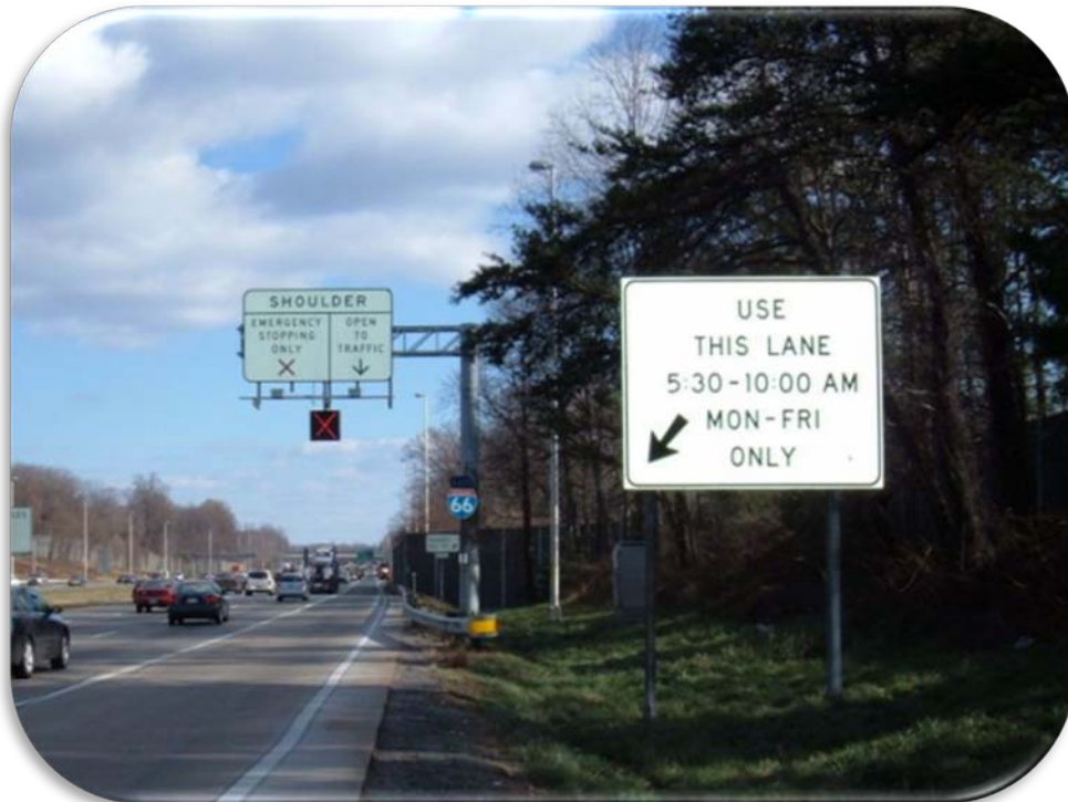
Figure 17. Photo. I-66 Hours of Use Regulatory Sign (Photo Courtesy of VDOT).
