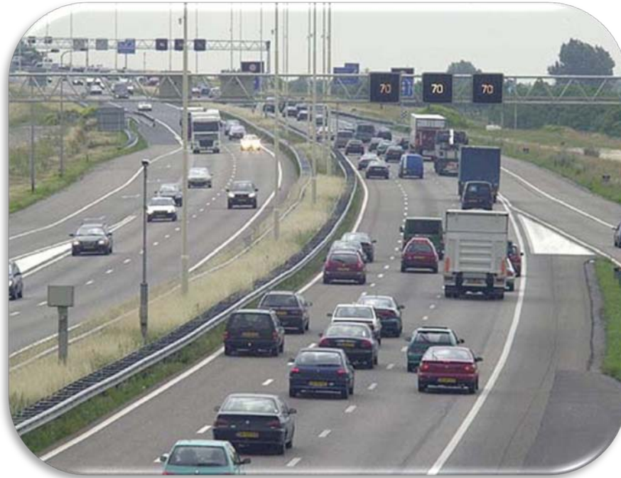
Figure 7. Photo. Plus Lane—The Netherlands. (1)
