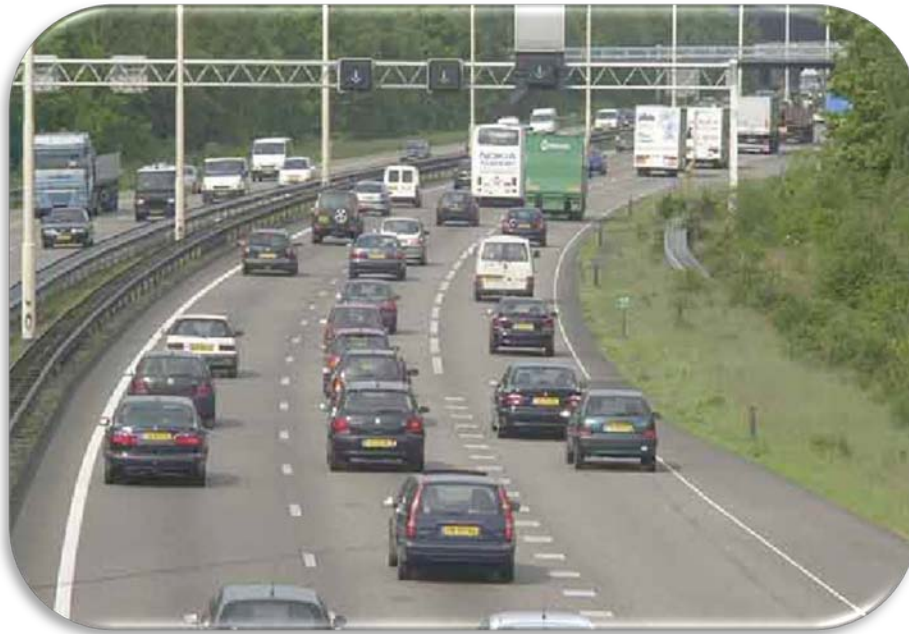
Figure 24. Photo. Temporary Right Shoulder Use—The Netherlands. (36)
